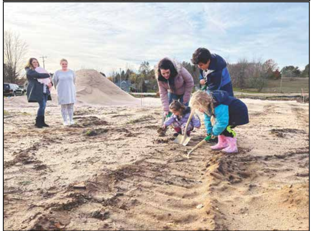
Above: The first energy-efficient duplex at Maple City Crossings is nearly ready for its occupants. Below: Emily Kelp and her children, Jayden, 8, Piper, 4, and Jenna, 2, “broke ground” in November 2021 on the affordable housing units as Kristina Eggeman, her eighth grade daughter Keely, and baby Vivian looked on. Both the Kelps and Eggemans will live here.
